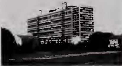
5. View of the half-finished Unite d'Habitation, Marseille, France, designed by Le Corbusier.
