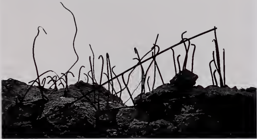
161. Shelled Bunker, Meschers #7 , 1950
